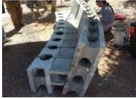
If you want to have a curved bench, lay out your pieces in a radius pattern that will form the bench and back to the desired curve before connecting the pieces with foam.
