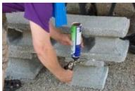
Fasten the bench legs with polyurethane foam adhesive – to reinforce the connections you may use pieces of rebar, dowels or bolts worked in to the connected material and anchored with the foam (If you use them, be careful not to extend them into any void spaces).
